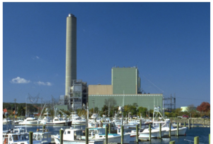
Canal Generating Station (Source: NRG)
